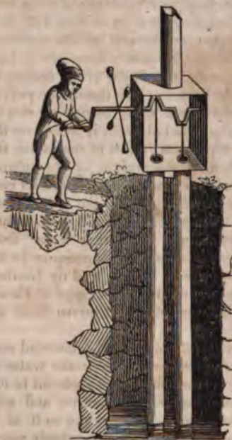
No. 128. Lifting Pump from Agricola.
